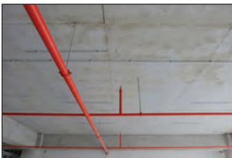
Check the slope of your piping to ensure that water cannot become trapped in branch lines
