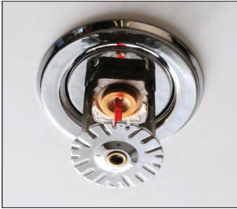
A typical automatic sprinkler head
